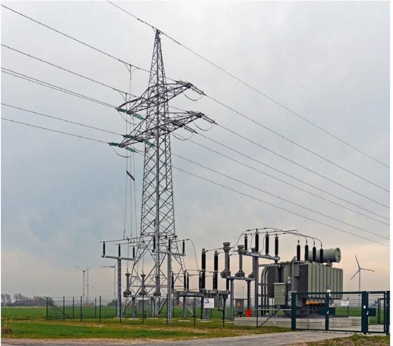
En example of a 72kV vacuum circuit breaker installation, copnnecting a renewable energy plant with a transmission network.
